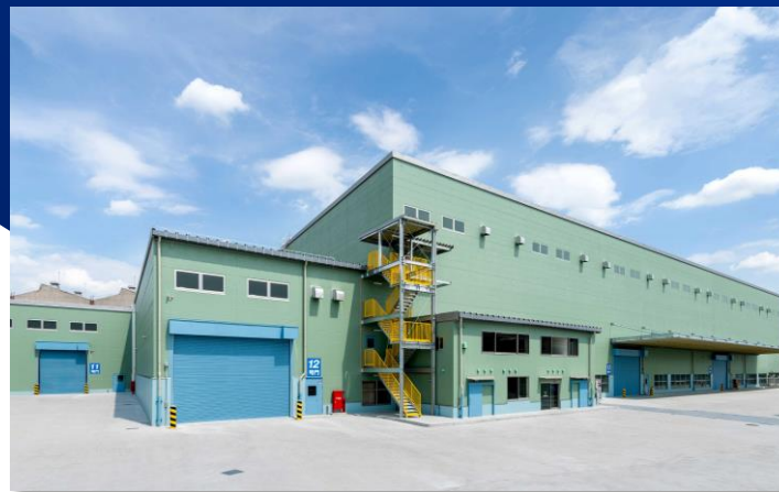
Kyoei Steel Ltd. Hirakata Office Product Warehouse
